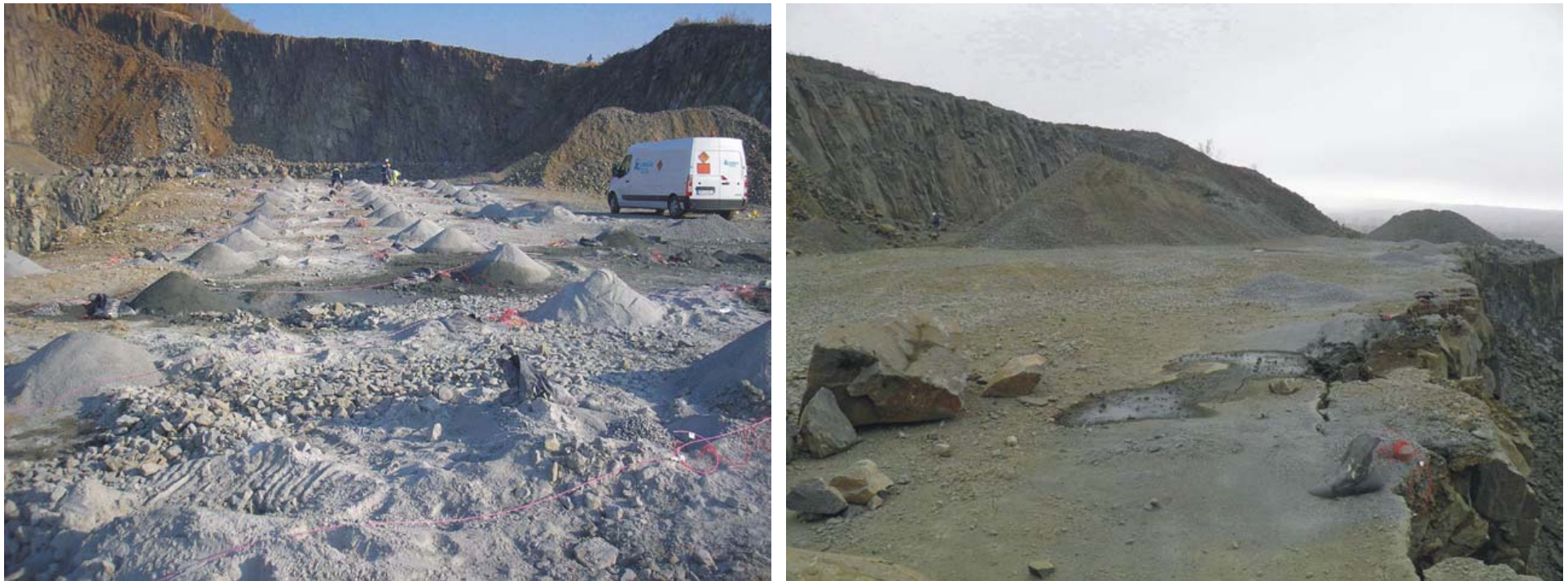
Fig. 4 Position of triplex drilling at bench blasting No. 357 and crown after blasting
