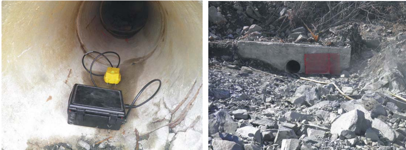
Fig. 9 Measuring position in a 0. storey, 10 m from the blast in the Maglovec quarry
