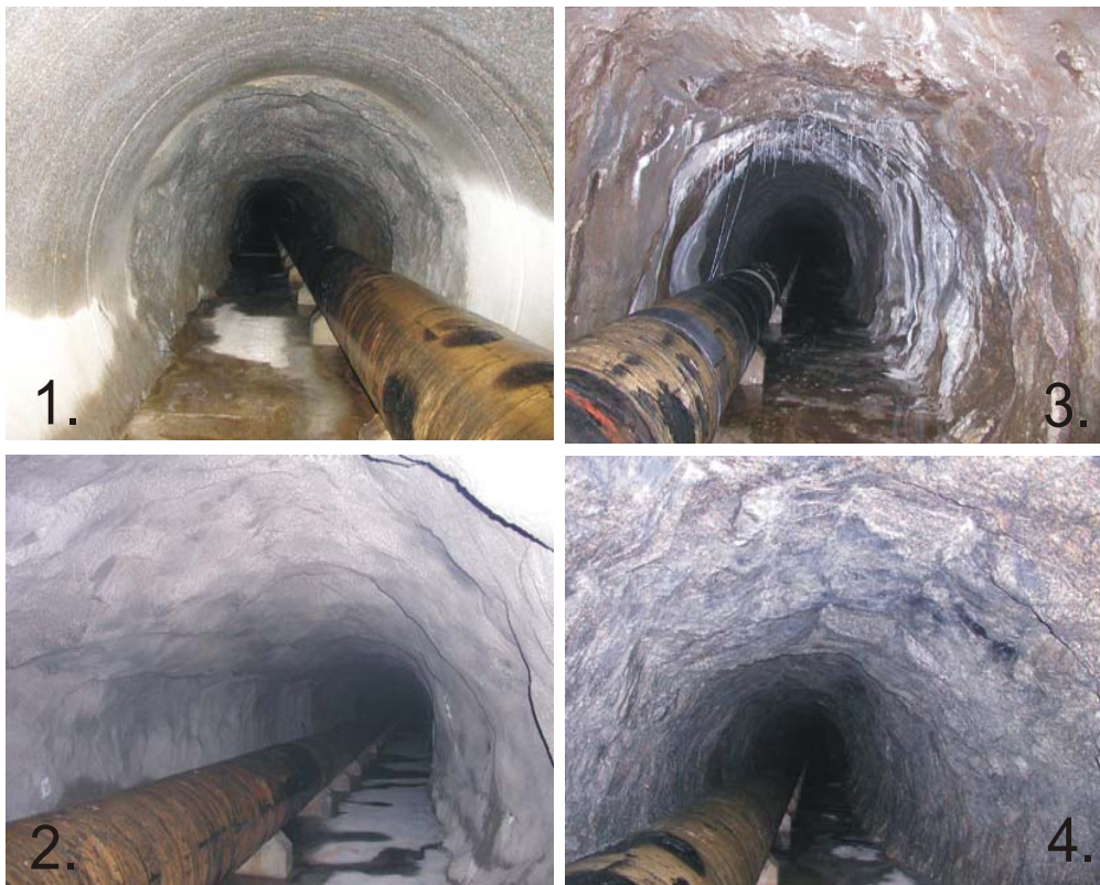
Fig. 1 Situation in the tunnel with combined blasted or bored parts [3]
