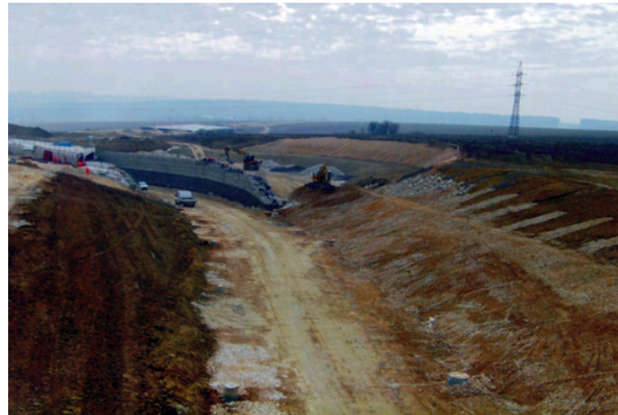
Fig.3 Supercharging of the slope and drainage edges (03/2011)
