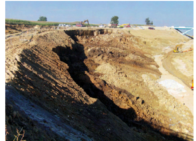
Fig.2 Disjointed wall of slope defect (09/2010)
