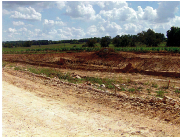
Fig.14 Slide at the right side cut
