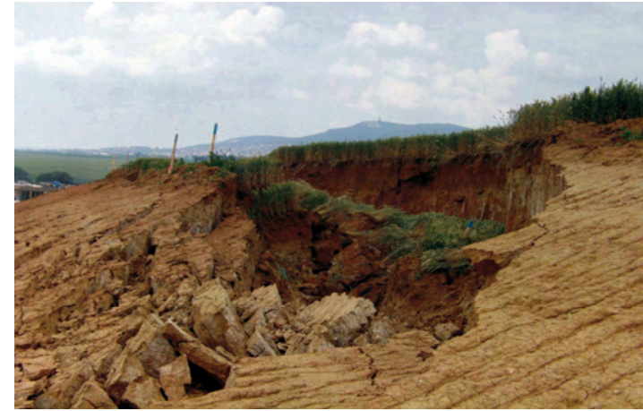
Fig.6 Separated wall– overlapping the construction site border
