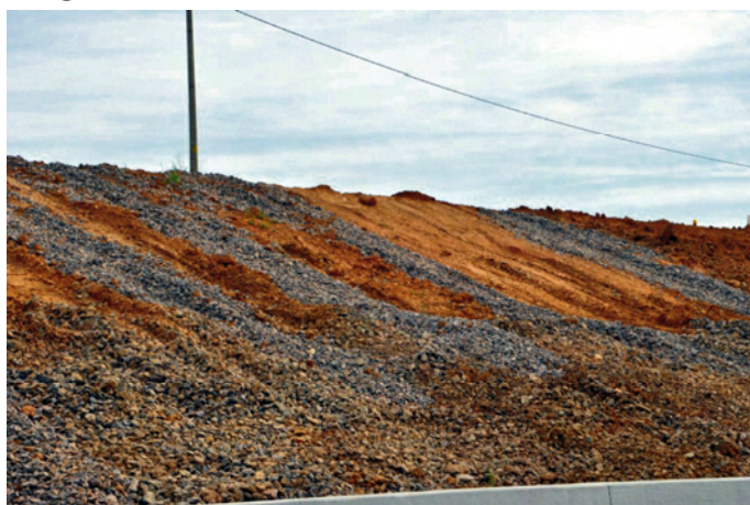
Fig.19 Drainage webs and surface drainage
