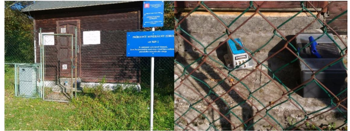
Fig. 5 The monitoring station MS2, water source MP-1 and Vibraloc measuring equipment including the three-component Vibraloc sensor on a special base on a concrete step in the entrance to the water source building
