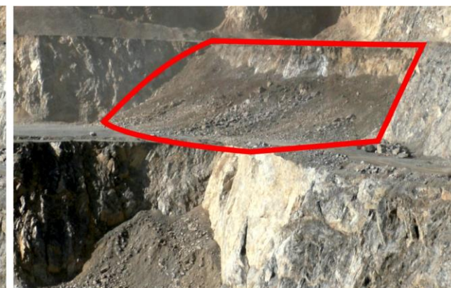
Fig. 10 Fresh rock after blasting of the quarry wall at the 3rd etage at bench blast No. 718
