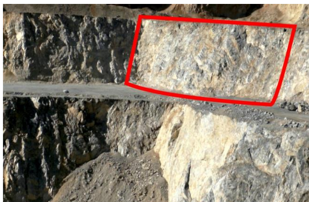
Fig. 9 View on the quarry wall in front of the bench blasting No. 718
