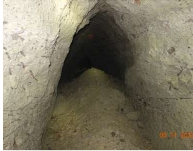
Fig. 14 CH1 mine – without a support Fig. 15 M2 corridor – a chimney shaft
